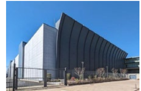
Mitaka Data Center EAST
