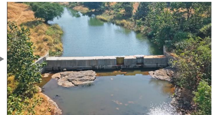
Completed water storage facility
